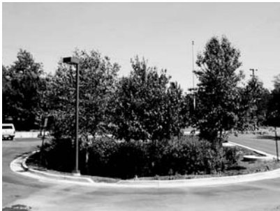
Bioretention systems can reduce the amount of storm water runoff generated by impervious surfaces, such as parking lots, that enters a CSS during wet weather.
