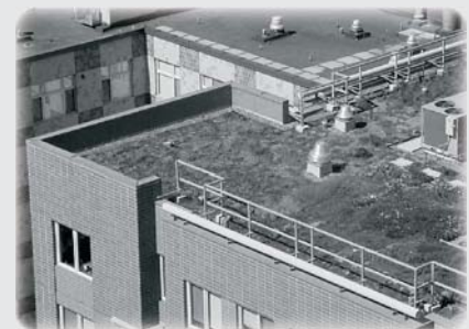
Photo: City of Portland Housing Authority
